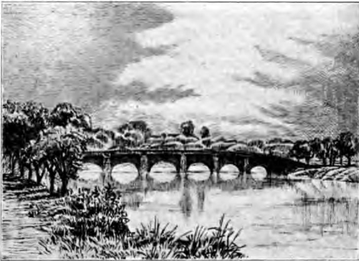
BRIDGE OVER THE COOUM NEAR GOVERNMENT HOUSE.
